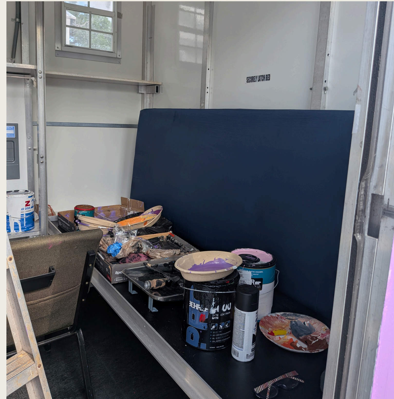
A hope cottage in Tampa under interior renovation.
